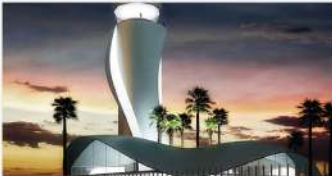
9 Fujairah International Airport, Fujairah
